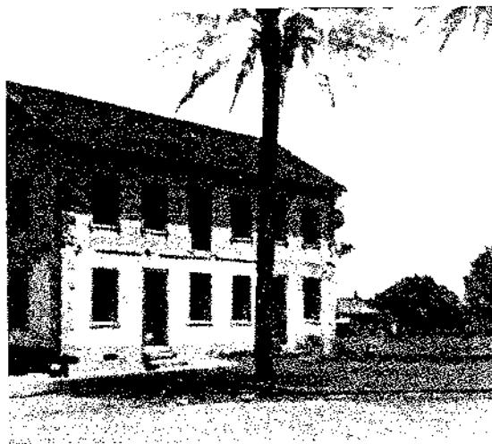
Garnier limestone building -- 1872
